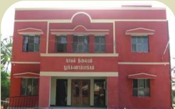
Police Station at Thookanampakkam Cuddalore Dist.
