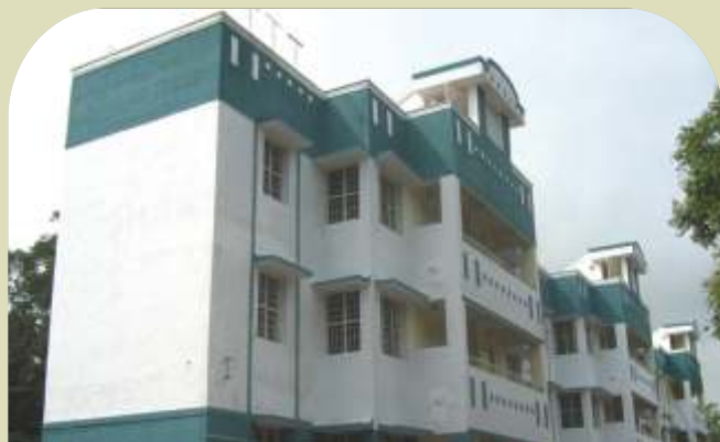
Jail Warder's quarters at Cuddalore
