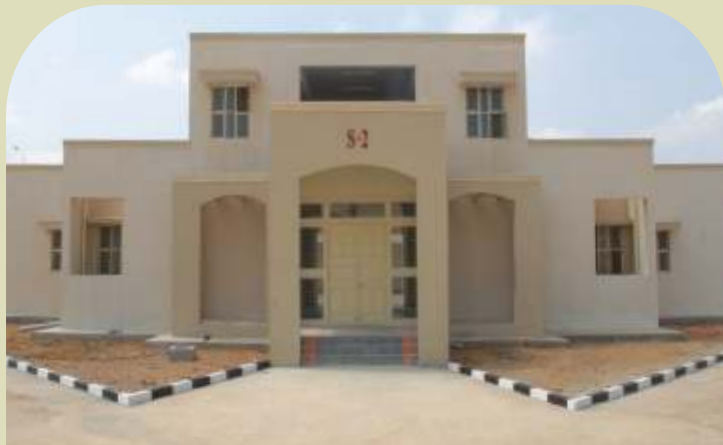
DSP's Accommodation Block
