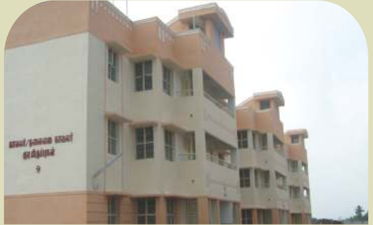
PC's / HC's quarters at Ulundurpet, Villupuram Dist.
