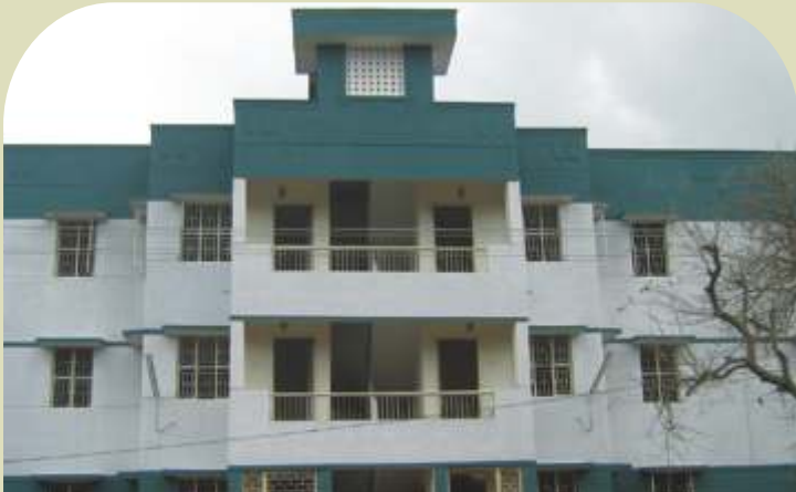
PC's / HC's quarters at Periyapalayam, Thiruvallur Dist.
