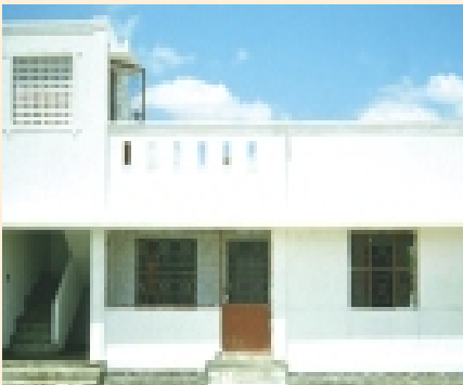
A view of Sub-Inspector's quarters at Mangalam
