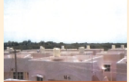
PVC Tank for each unit
