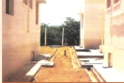
Sullage drain arrangements
