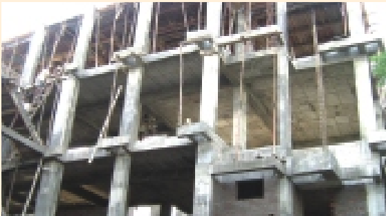
Forensic building in Progress
