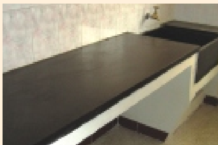
PC's / HC's quarters at Saidapet Kitchen arrangements
