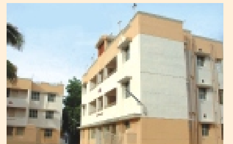
Palayamkottai Rs. 42.11 lakhs
