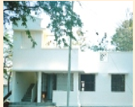
A view of Inspector's quarters at Sathyamangalam
