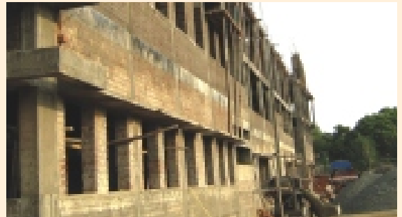
Forensic building in Progress
