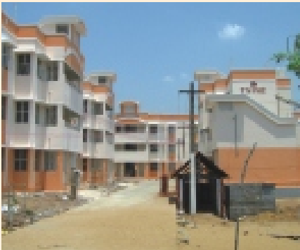
13 PC's / HC's quarters for Railway Police at Kumbakonam
