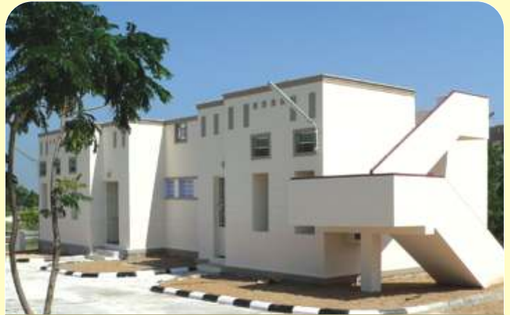
Dormitory , Thiruvannamalai Dist.
