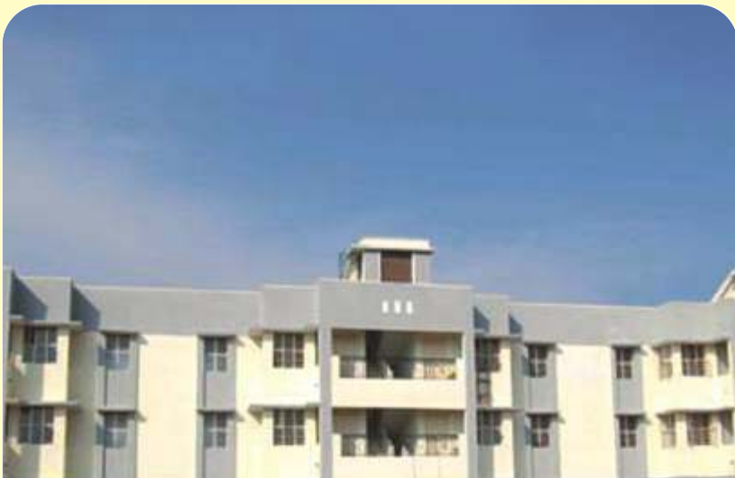
Firemen's Quarters at Pettai - Tirunelveli
