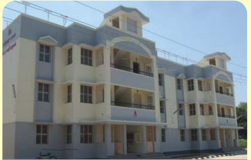
Firemen's Quarters at Rajapalayam
