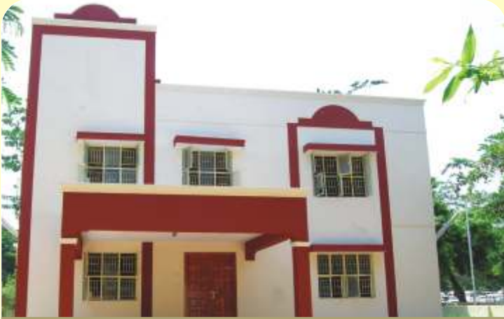
In Service Training Centre, Pudupet, Chennai
