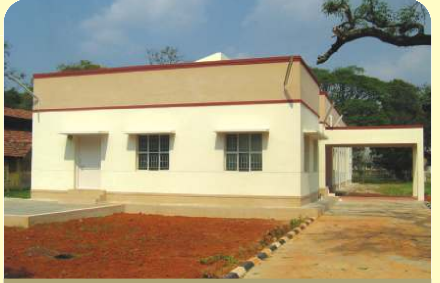
Barracks at Avadi
