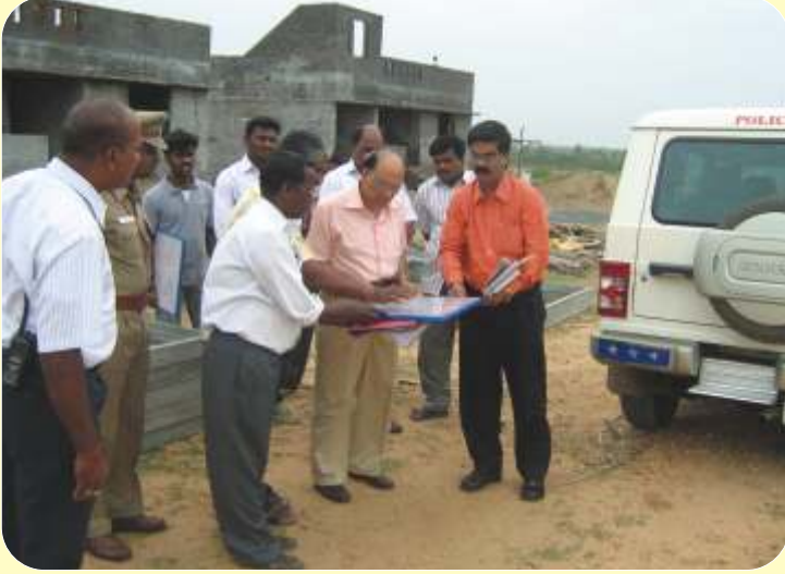
The DGP cum CMD/TNPHC has inspected the construction work of 2 INS, 3 SI and 60 PC/HC quarters at Tiruvannamalai on 12.06.08
