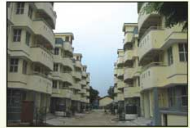
104 PC's / HC's quarters at Dhakshinamoorthy Koil Street, Chennai
