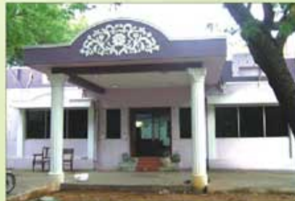
Modern Control Room at Trichy
