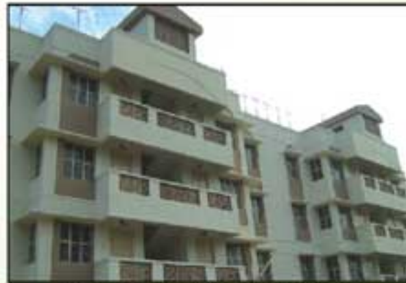
156 PC's / HC's quarters at Mambalam, Chennai
