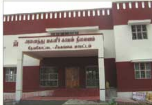
AWPS at Devakottai, Sivagangai District
