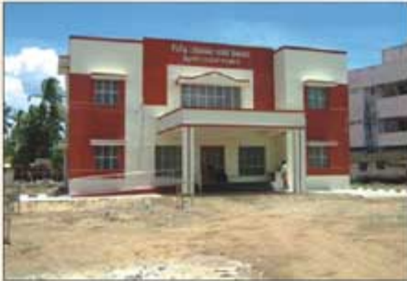
Police Station at Palakarai, Trichy District
