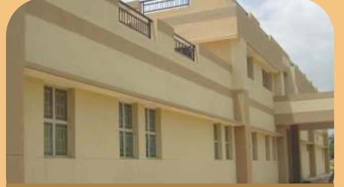
A View of AR building at Krishnagiri
