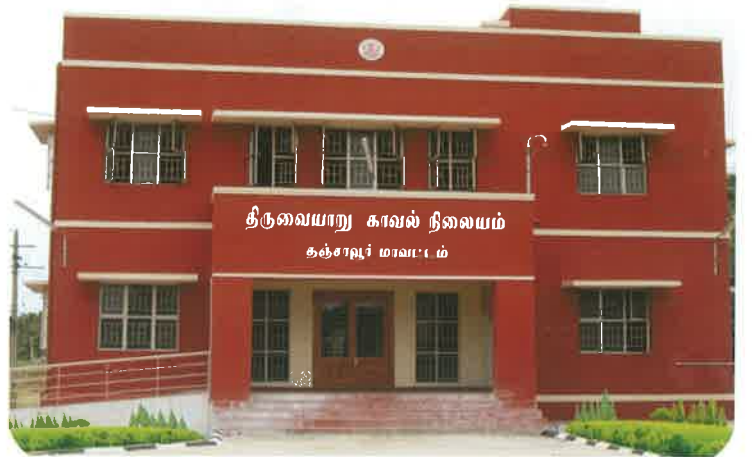
Police Station, Thiruvaiyaru, Thanjavur District
