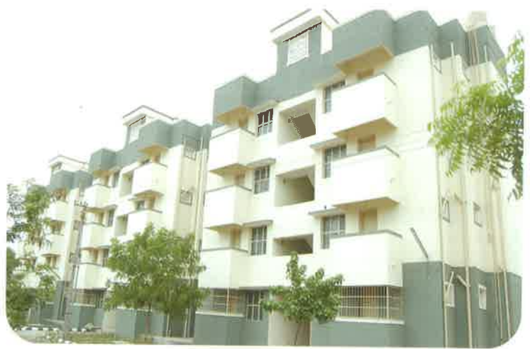
PC/HC Quarters, AR Madurai City, Madurai
