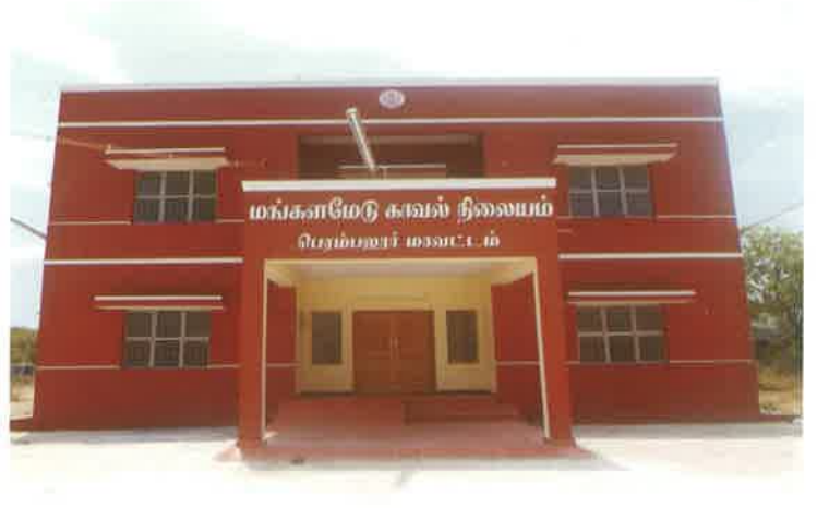
Police Station, Mangalamedu, Perambalur District
