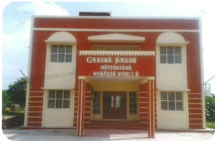
Police Station, Acharapakkam, Kancheepuram District
