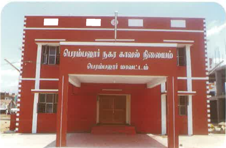
Police Station, Perambalur, Perambalur District
