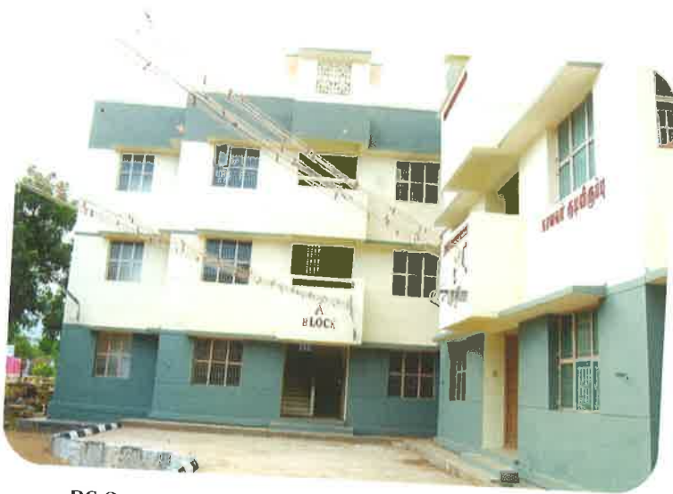
PC Quarters at Puliyanakudi, Tirunelveli District
