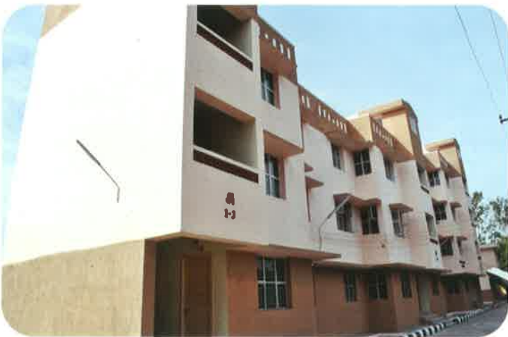
SI & PC/HC Quarters at Olakkur in Villupuram District
