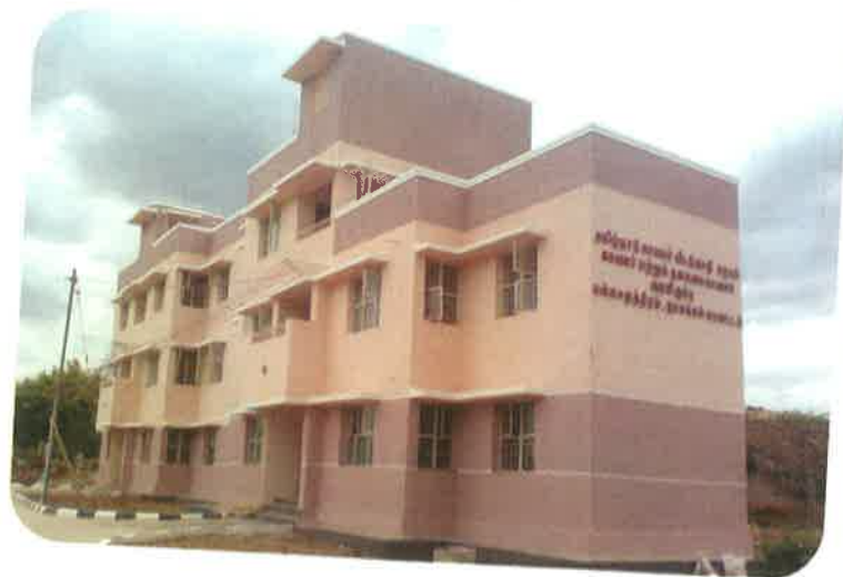
PC/HC Quarters at Mallasamudram in Namakkal District
