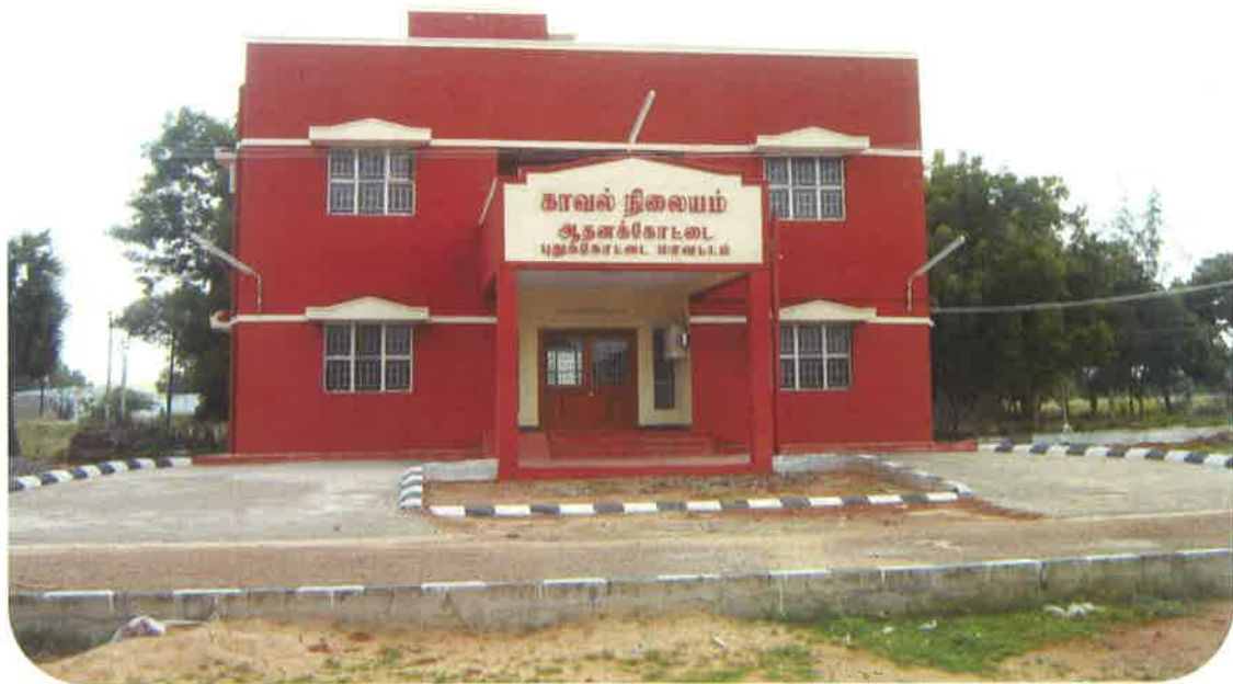
Police Station, Athanakottai, Pudukottai District
