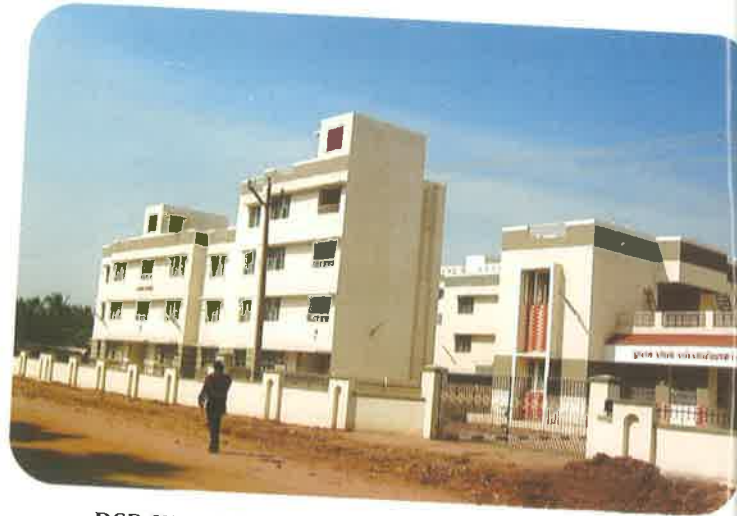
DSP, INS, SI, PC/HC Quarters at Avadi, Chennai
