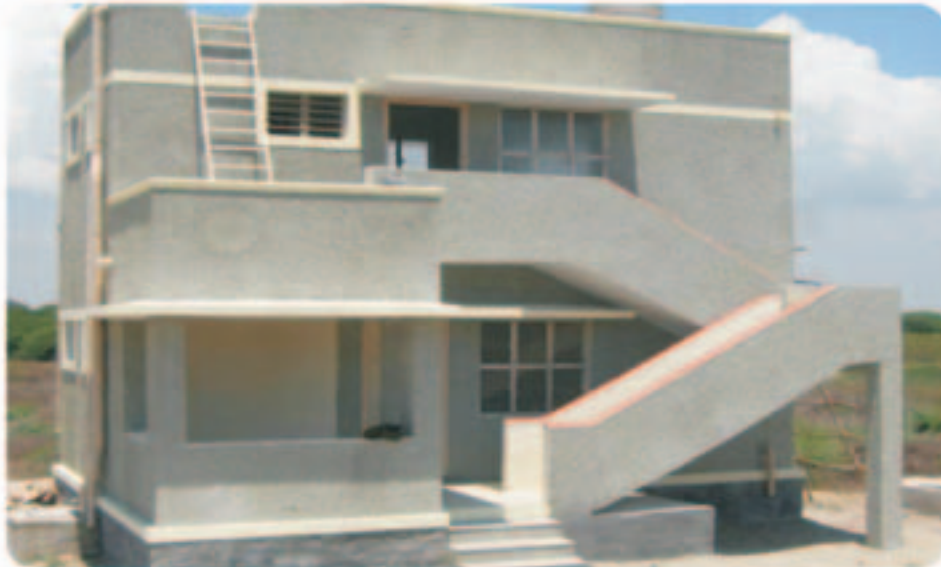
Check Post, Patinamaruthur, Madurai Dist.
