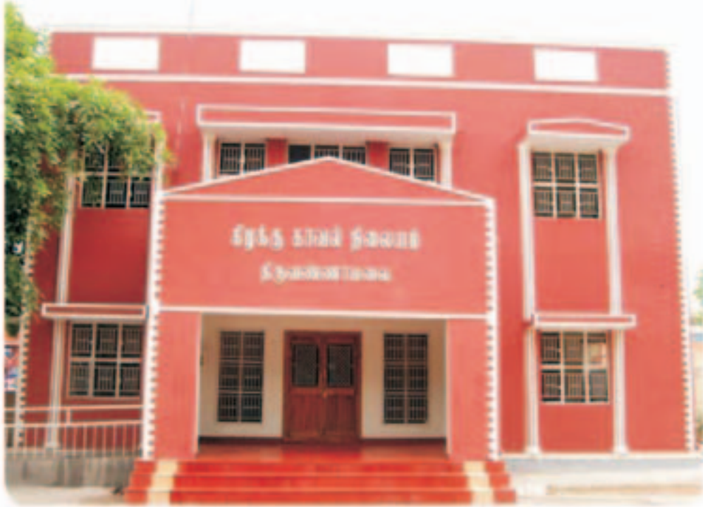
Rural Police Station, Thiruvannamalai East, Thiruvannamalai Dist.
