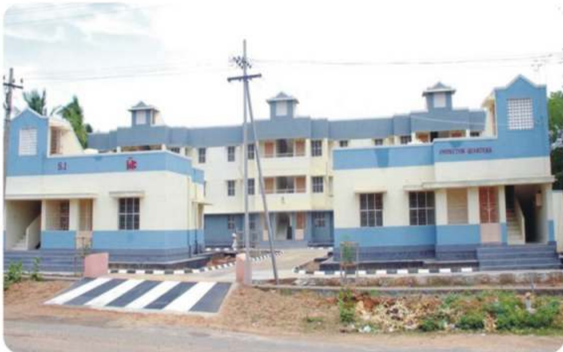
Sub Inspector Quarters, Viralimalai, Pudukottai Dist.
