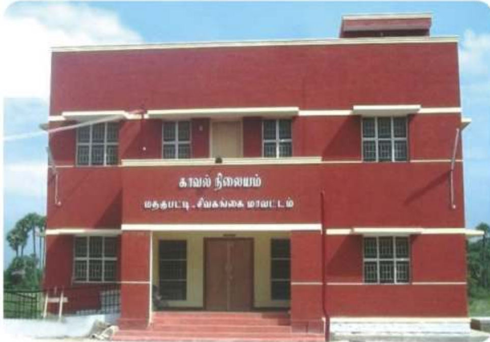
Police Station, Mathagupatty, Sivagangai Dist.
