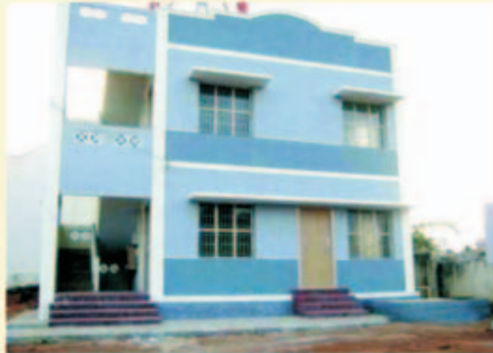
Repeater Station, Kanniyakumari Dist.
