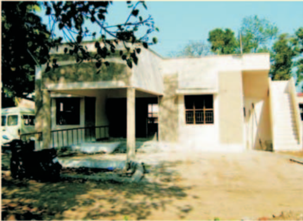
SBCID Office Building, Cuddalore Dist.
