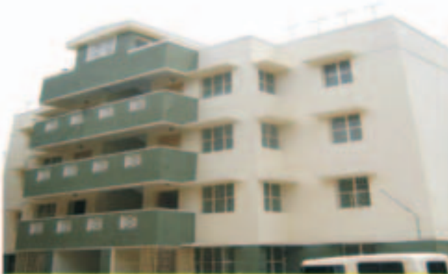
PC / HC Quarters, Desigar Street, Chennai
