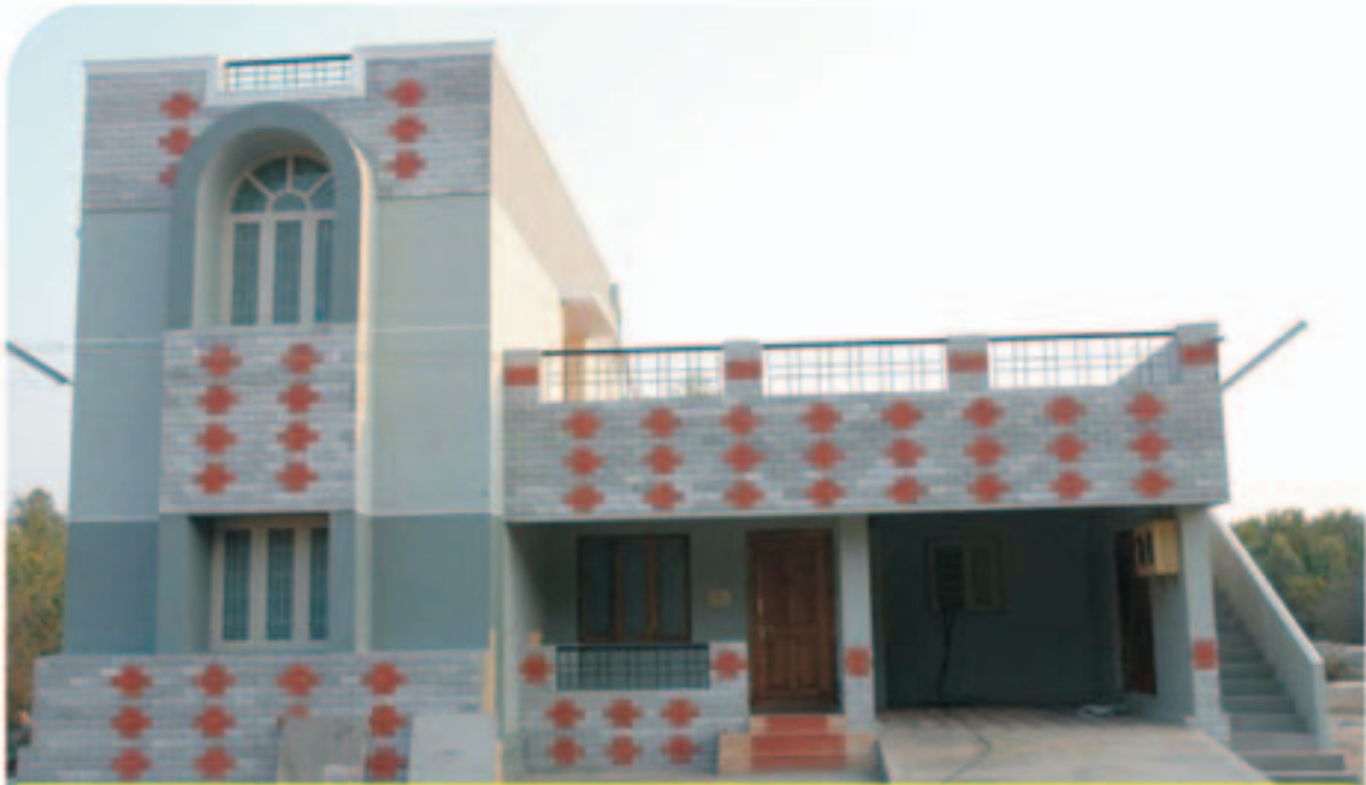
DSP Quarters, Bargur, Krishnagiri Dist.
