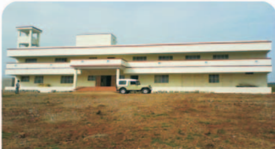
Dormitory, Othivakkam, Chennai
