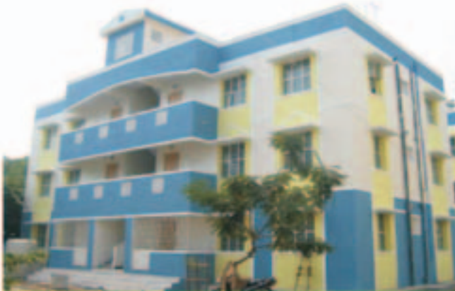
Ins. Quarters, Pudupet, Chennai
