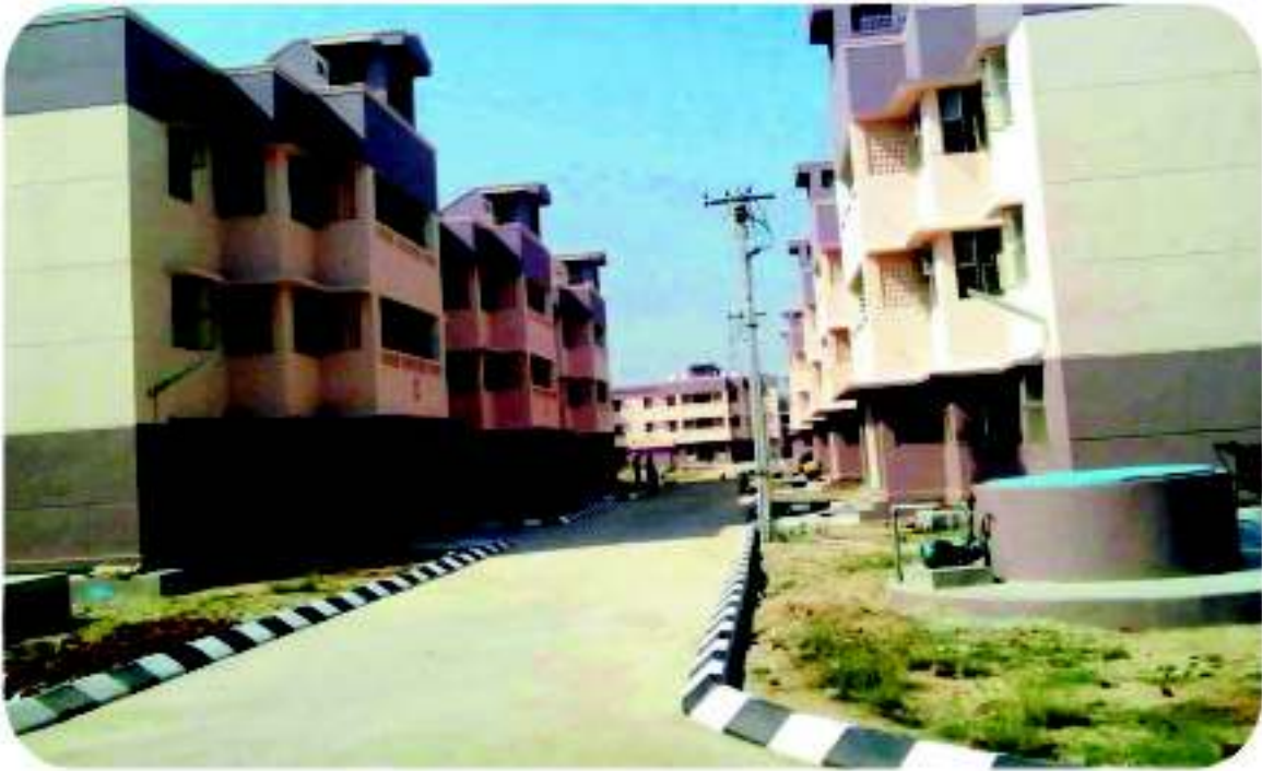
PC / HC quarters at Ramanathapuram A.R.
