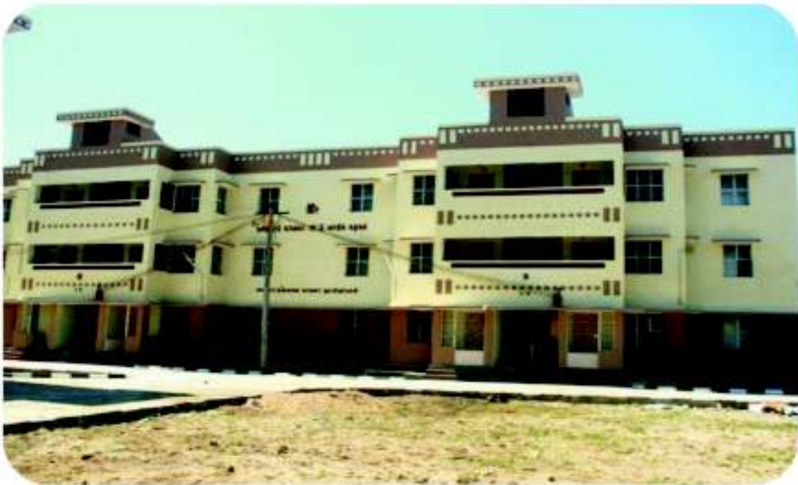
PC / HC quarters at Kandachipuram, Villupuram Dist.
