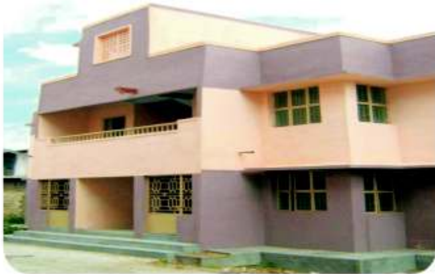
Firemen Quarters at Udumalpet, Coimbatore Dist.
