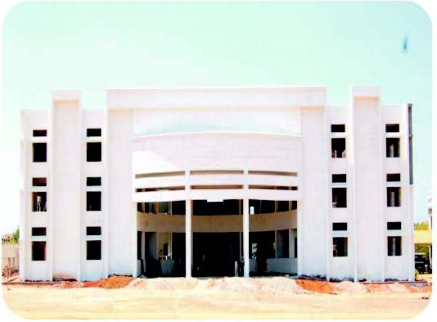
City Police Office at Tirunelveli (under construction)
