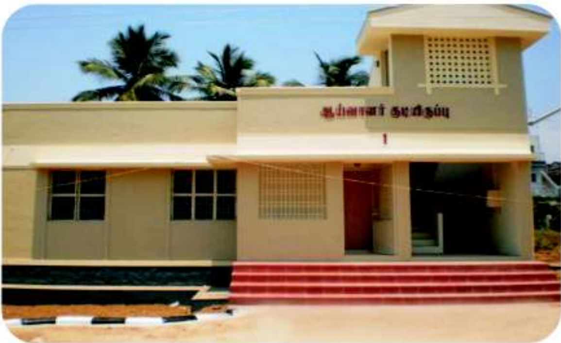
Inspector quarters at Jolarpet, Vellore Dist.
