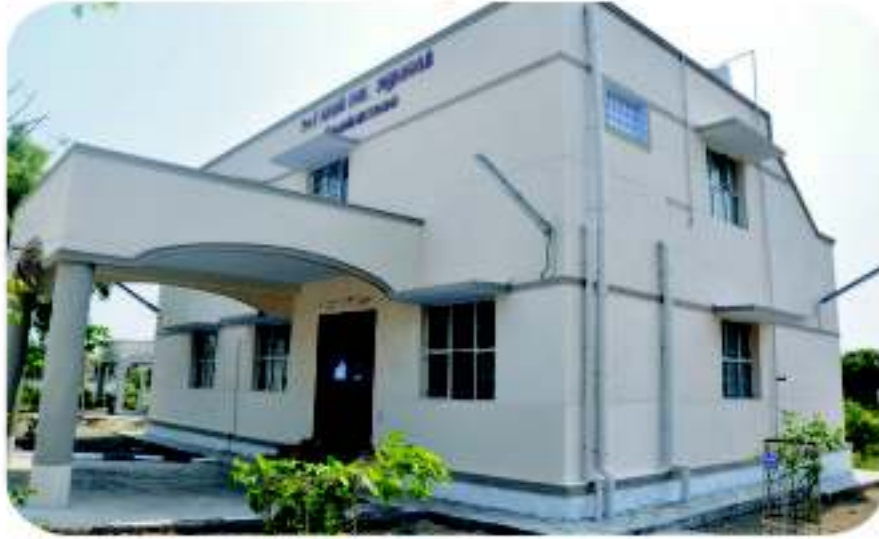
Home Guard Office at Thiruvannmalai Dist.
