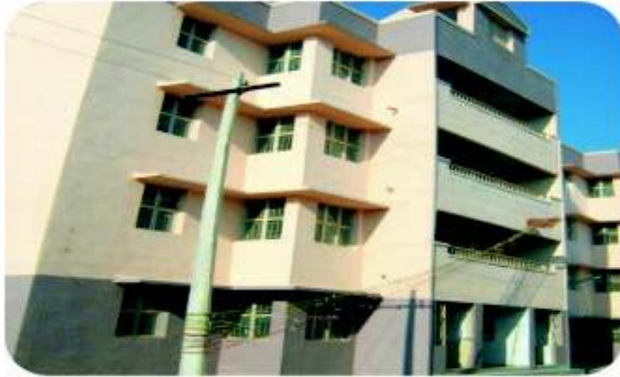
Firemen Quarters at Udumalpet, Coimbatore Dist.
