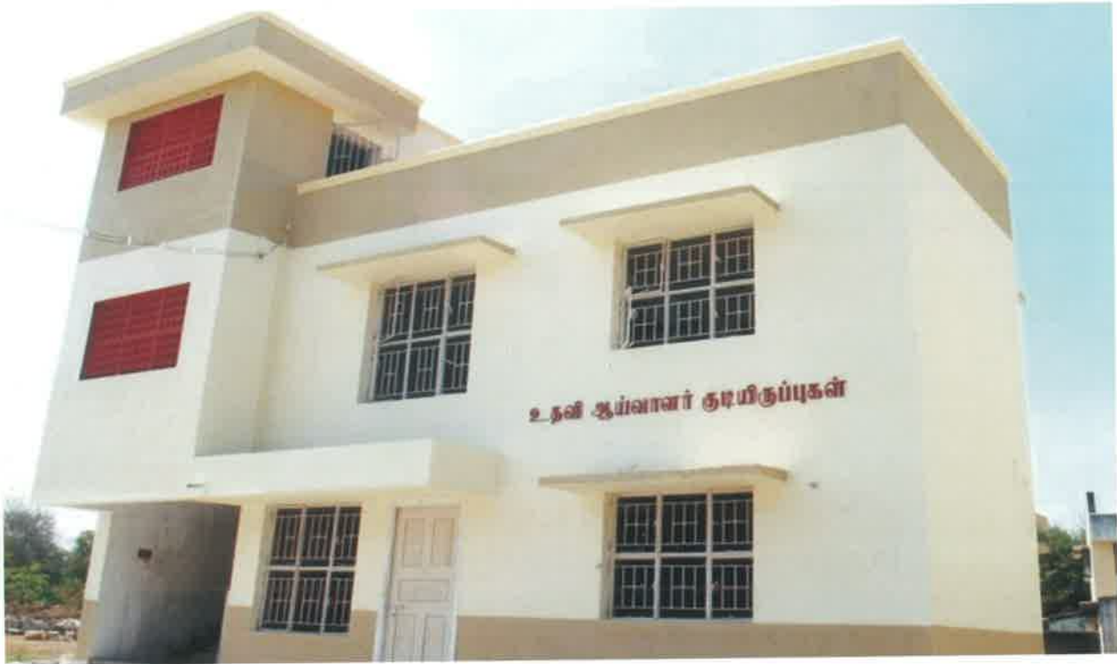
Sub Inspector Quarters, Mailam, Villupuram Dist.
