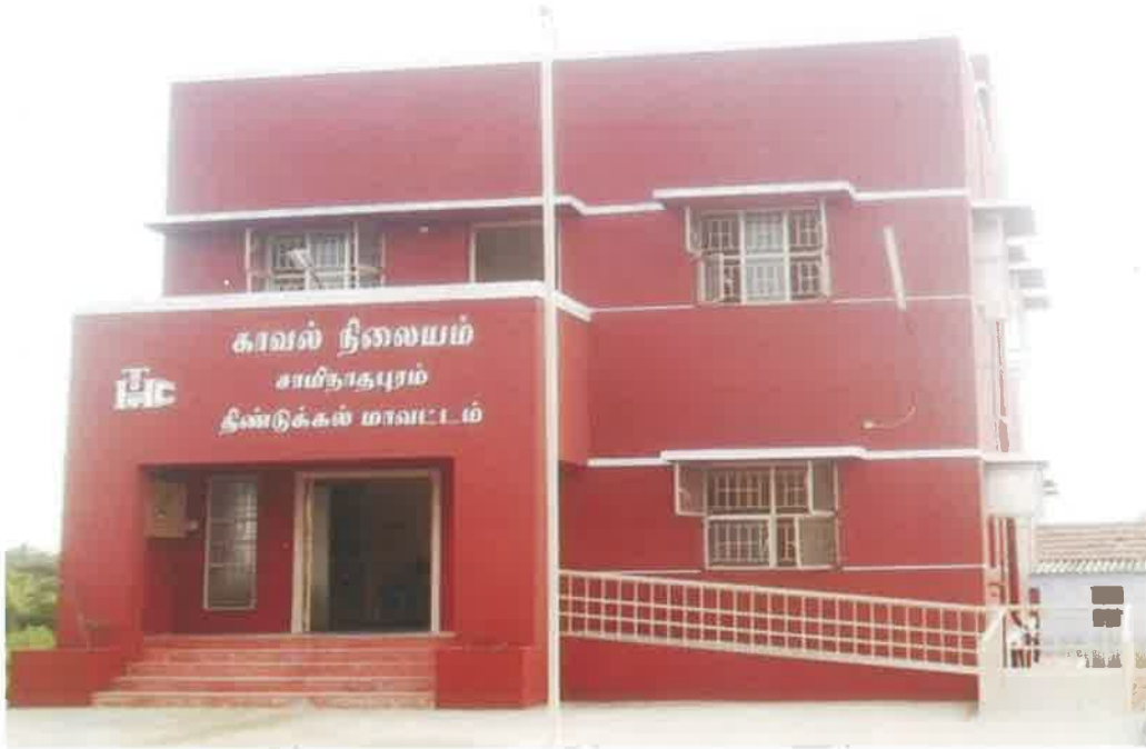
Police Station, Saminathapuram, Dindigul Dist.
