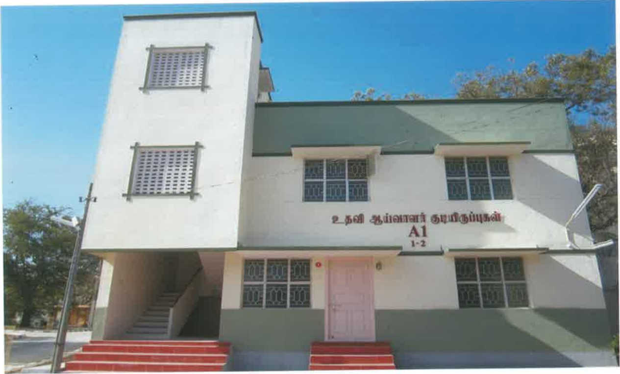
SI Quarters, Thiruvannamalai Group I, Thiruvannamalai Dist.
