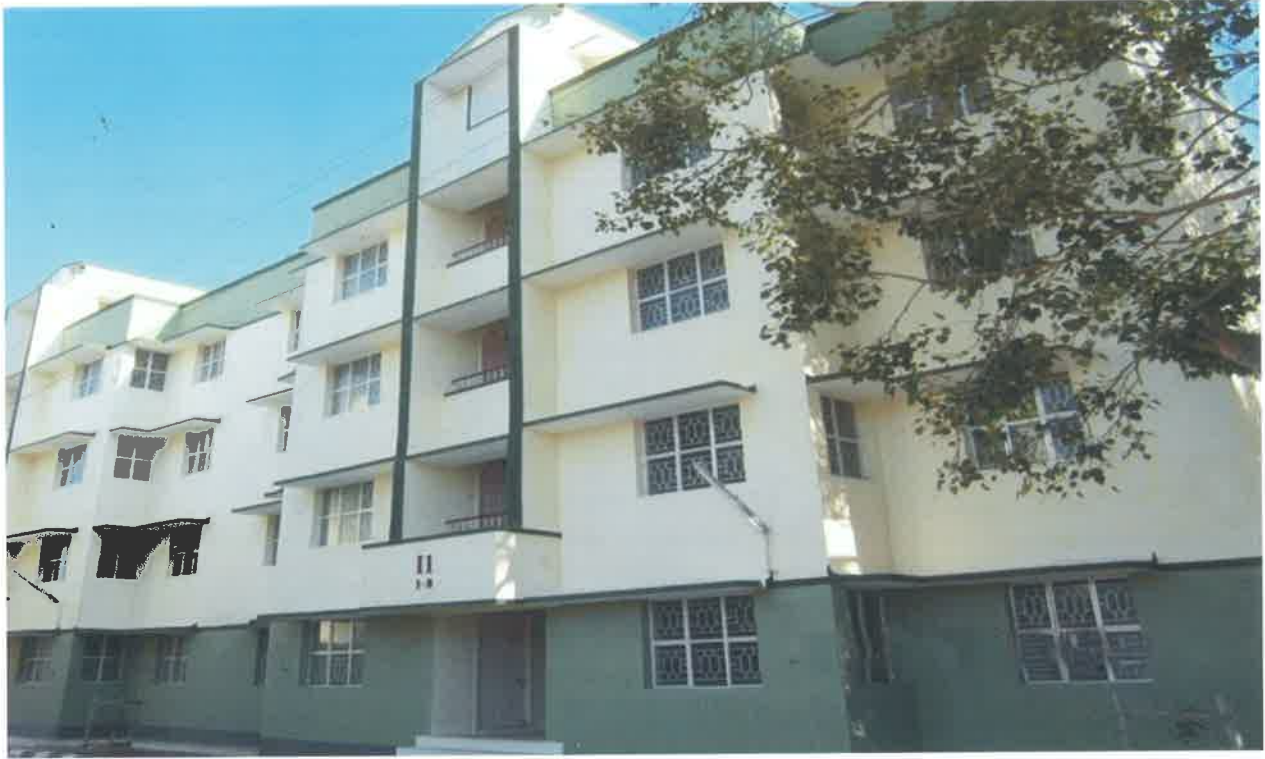
PC / HC Quarters, Thiruvannamalai Group IV, Thiruvannamalai Dist.
