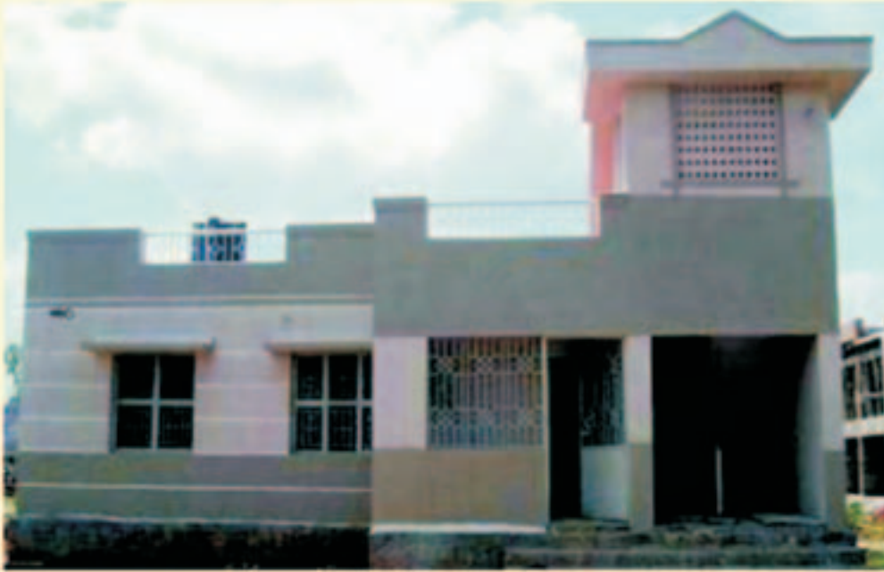
Inspector Quarters, Denkanikottai, AWPS & P.S. Krishnagiri Dist.
