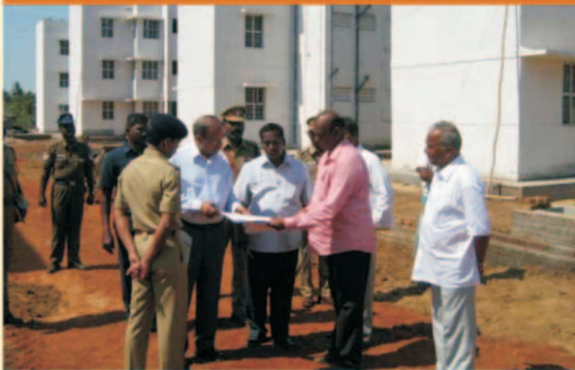
Inspection of Thiruvannur AR Quarters, Trichy by the Managing Director / TNPHC
