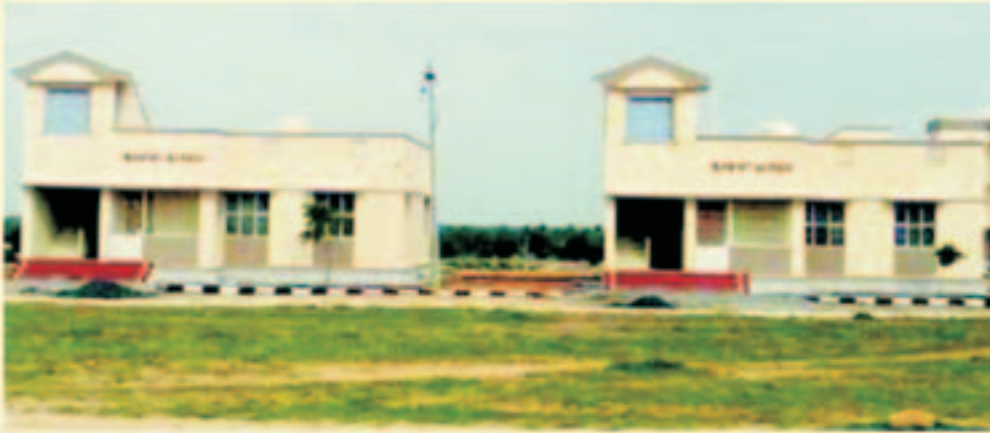
Inspector Quarters, Thiruvannamalai Town, Thiruvannamalai Dist.
