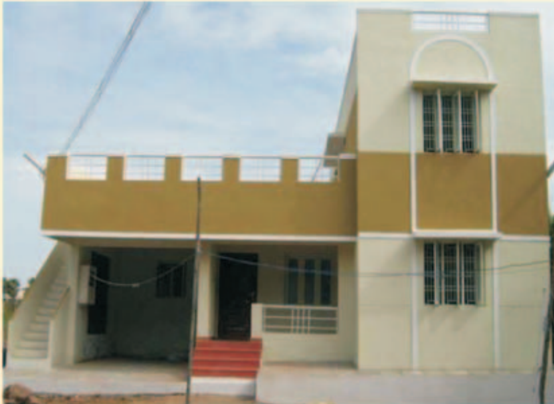
DSP Quarters, Thiruvarur Dist
