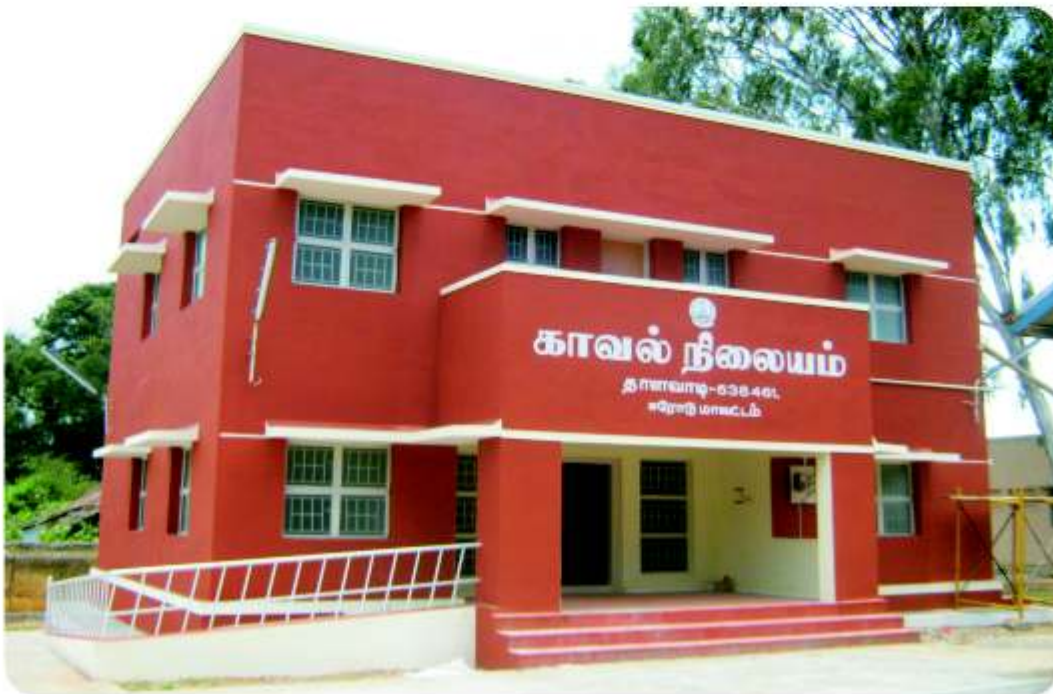
Police Station, Thalavadi, Erode Dist.
