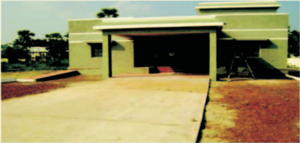
Marine Police Station, Manalmekudi, Pudukottai Distt.
