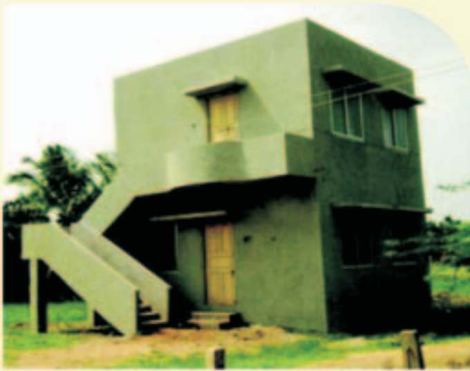
Check Post, Krishnagipattinam, Pudukottai Dist.
