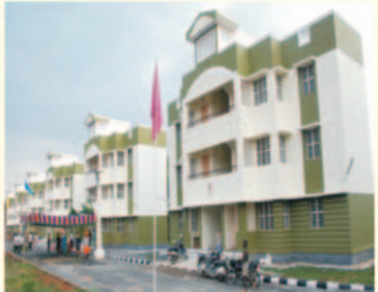
A view of Prison Warders Quarters at Vellore
