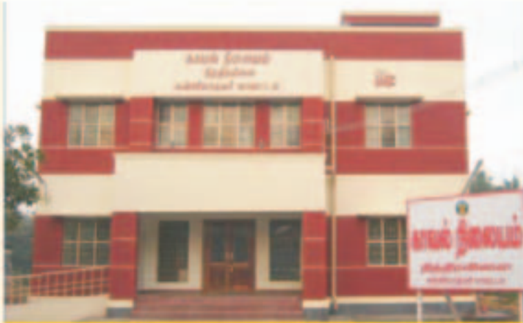
Rural Police Station, Nithiravillai, K.K. Dist.
