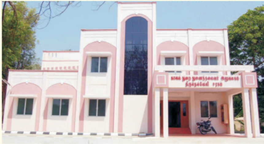
DIG Range Office, Tirunelveli Dist.
