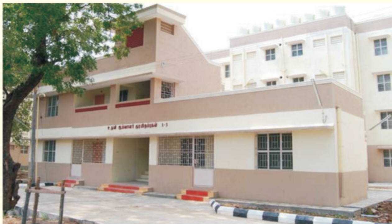
SI Quarters, Villupuram Town, Villupuram District
