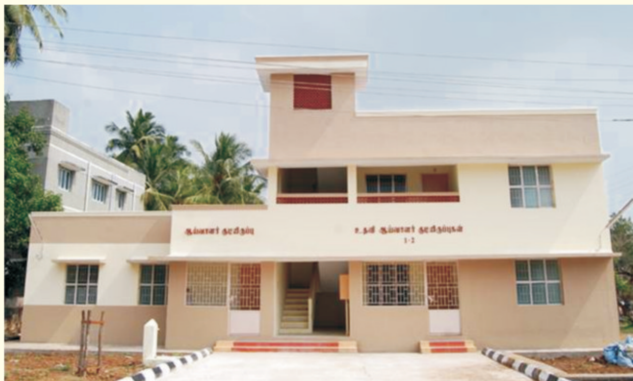
Inspector and SI Quarters, Villupuram Taluk, Villupuram District
