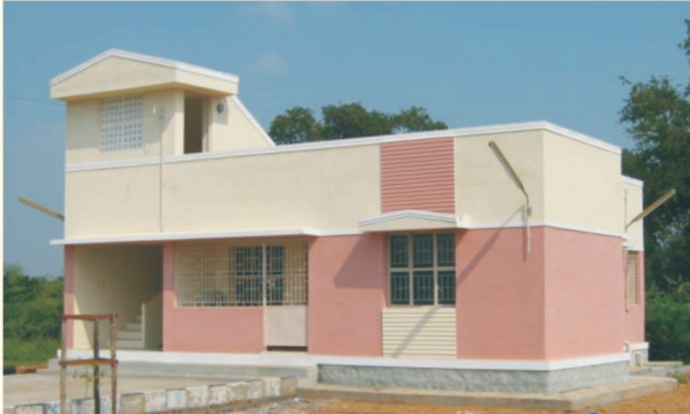
Deputy Jailor Quarters, Central Prison, Trichy Dist.
