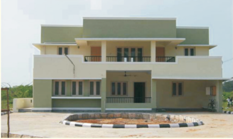
Superintendent Quarters, Central Prison, Trichy Dist.
